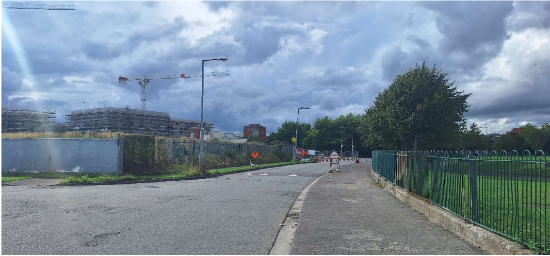
Figure 1.6 view from Barnville looking northwards with Site 5 on the left and Cherry Orchard Park on the right. Phase 1 of the Cherry Orchard Point Development can be seen under construction in the middle distance.
