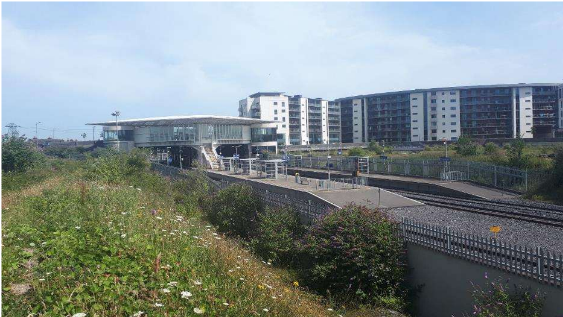
Figure 1.5 View of the southern boundary, railway cutting and Cherry Orchard railway station, with the Concert and Crescent buildings in the background.
