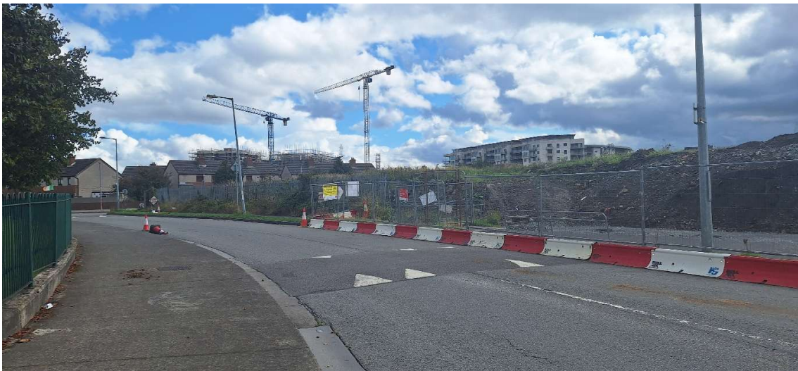
Figure 1.7 This view is taken from close to the junction of Barnville and Cedarbrook Way looking southwards. Site 5 is on the right, and the railings of Cherry Orchard Park are on the left. The roadworks in the foreground are associated with Cherry Orchard Point Phase 1. The site under construction in the middle distance is the LDA scheme Park West Pointe.
